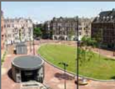
The Staringplein in Amsterdam has an automated underground car park.
