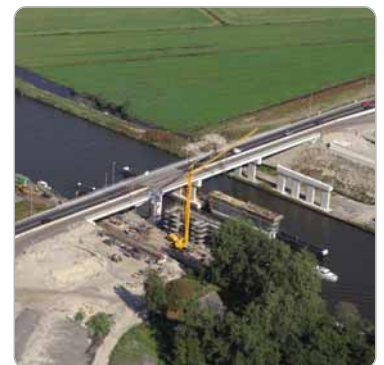
Fonejacht bridge, N31 The access ways have an MSWI bottom ash foundation.
