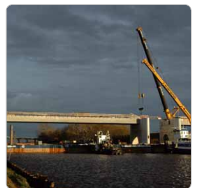
Eibersburen bridge The bridge with the longest pre-stressed girder in the Netherlands.
