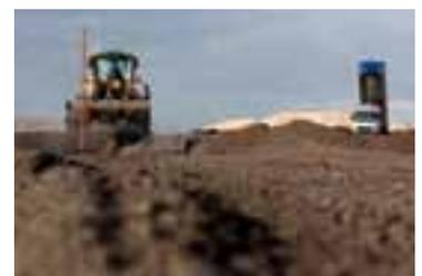
The A50 between Ewijk and Valburg is widened and the interchanges are changed dramatically. At the interchange Ewijk a completely new exit of Den Bosch to Nijmegen is developed where a lot of sand is needed. Sand is expensive, scarce and finite as a raw material. It was therefore decided to use incineration ash from the waste power plants, a secondary raw material.
