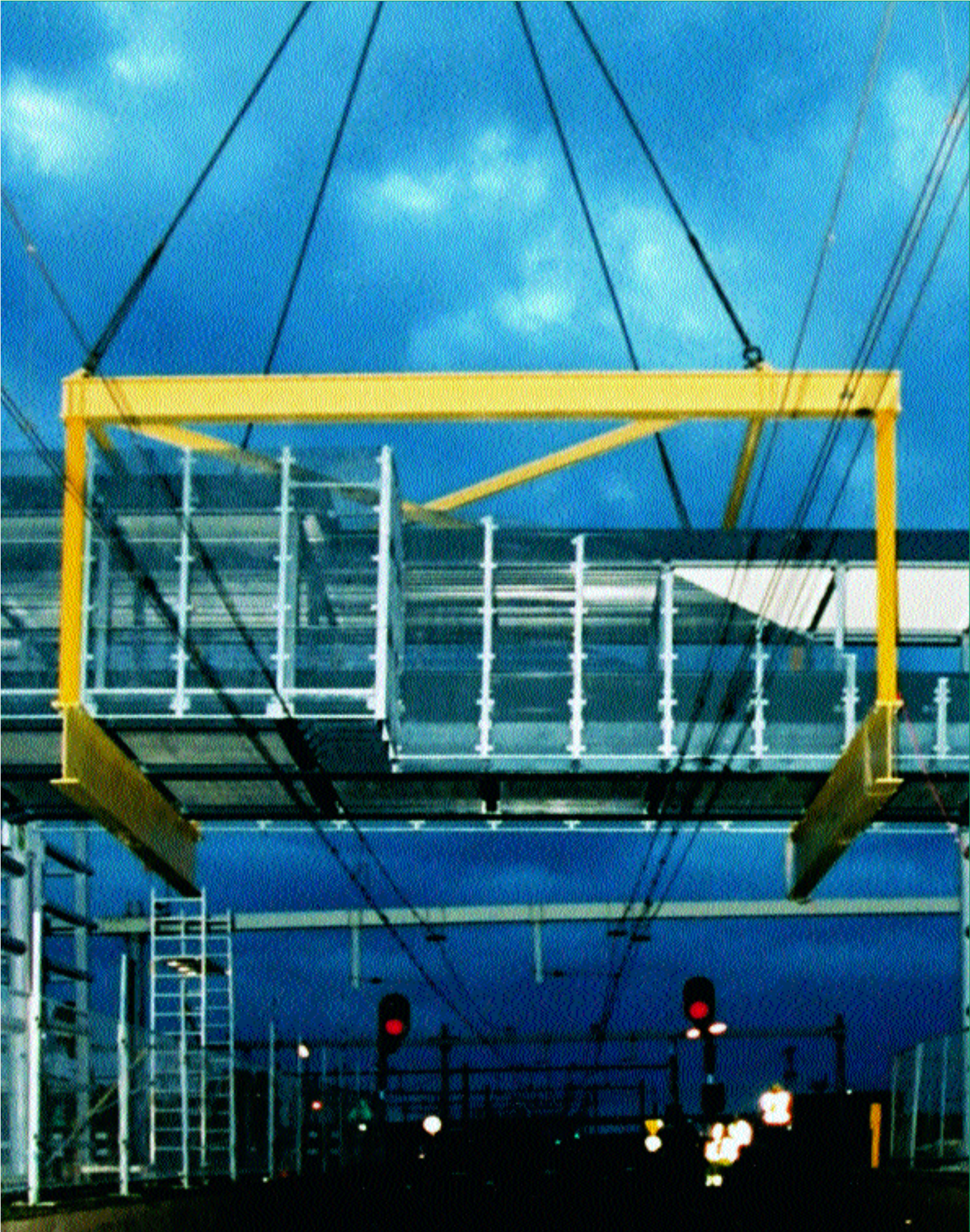
At Lage Zwaluwe station, the high-speed rail line runs parallel to existing intercity tracks. The glass footbridge gives passengers safe access to the platforms.
