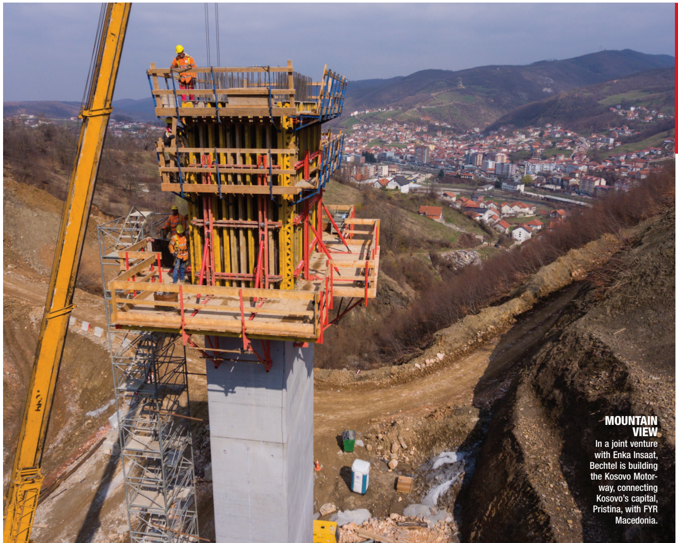
PHOTO COURTESY OF BECHTEL
